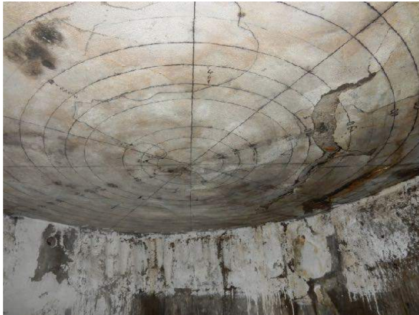
The map room of Yamamoto's bunker indicating distance rings and bearings of different locations from Rabaul
