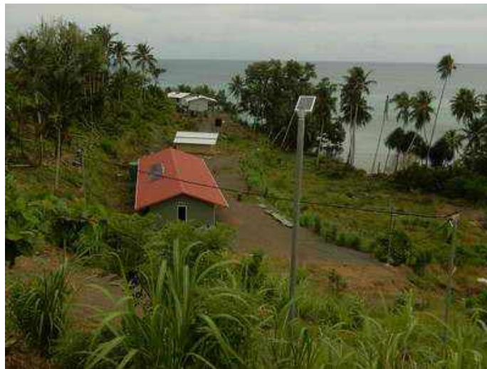
The New Girls' Dorm with Solar Electricity and Water.
