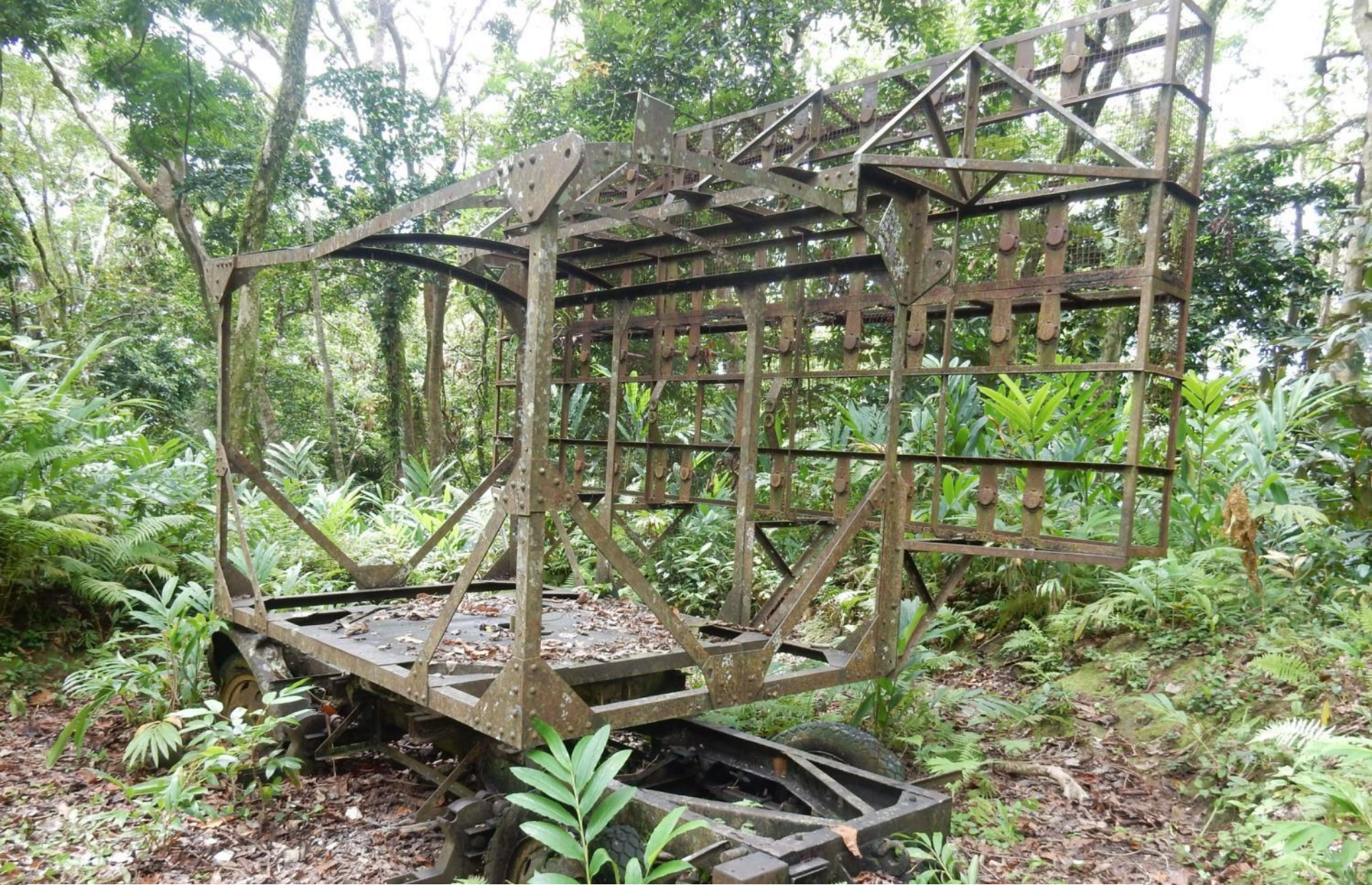
Radar Installation, Nila Ridge Trail Shortlands
