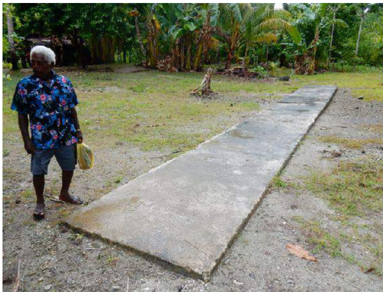
Nicely and an unknown concrete foundation in the WWII Naval Hospital area.
