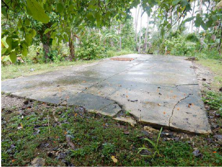
A concrete foundation for one of the WWII Naval hospital buildings on Pao Island.
